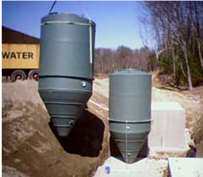
FIGURE 5 Typical Bioclere Filter Unit
