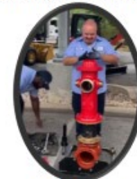
Fire Hydrant Demo
