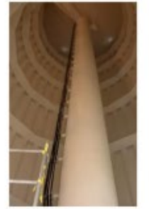
Inside the Elevated Water Storage Tank
